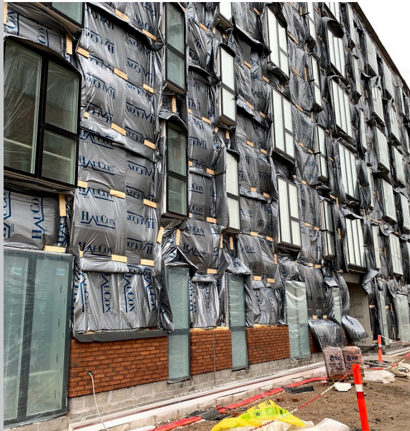
Combitherms winter mats with HauCons own logo are developed to protect the building from frost, rain, heat and sunlight. The winter mats are used to cover newly cast foundations and other forms of masonry, casting and earthwork.
